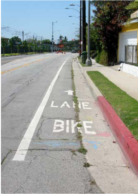
Substandard Bike Lane - Image shows minimum width of lane including rather than excluding the gutter pan. Source: www.betterbike.org
