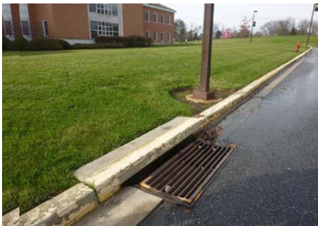
Un-Safe Drainage Grates
